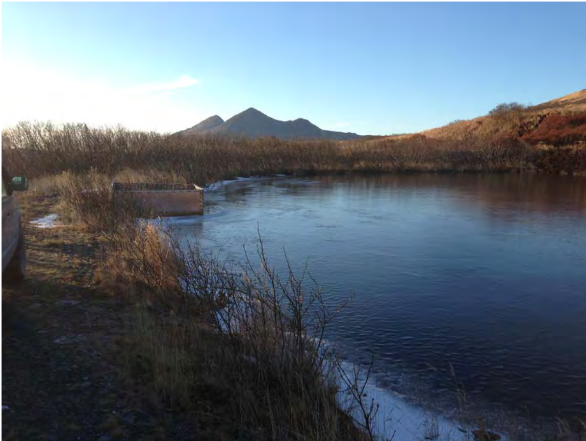
Akhiok's raw water reservoir
