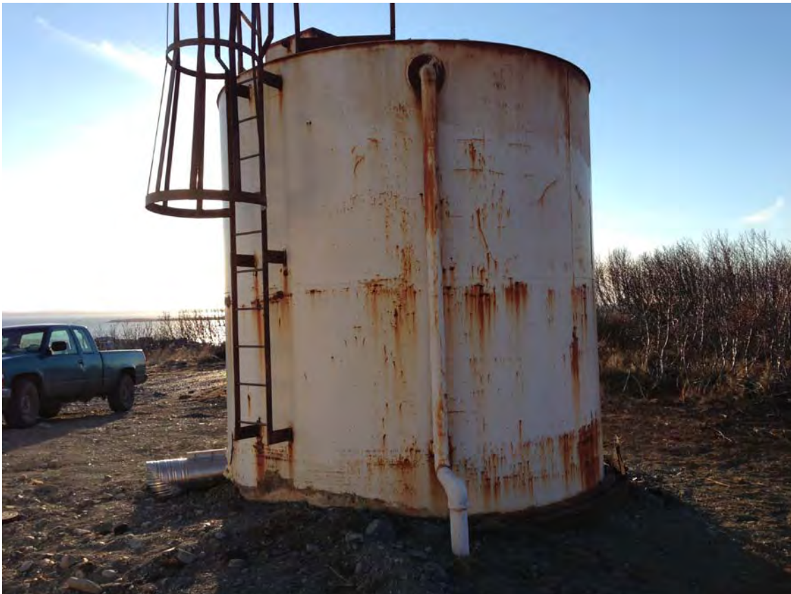
One of Akhiok's 10,000 Gallon WSTs (the other WST is directly behind this one)
