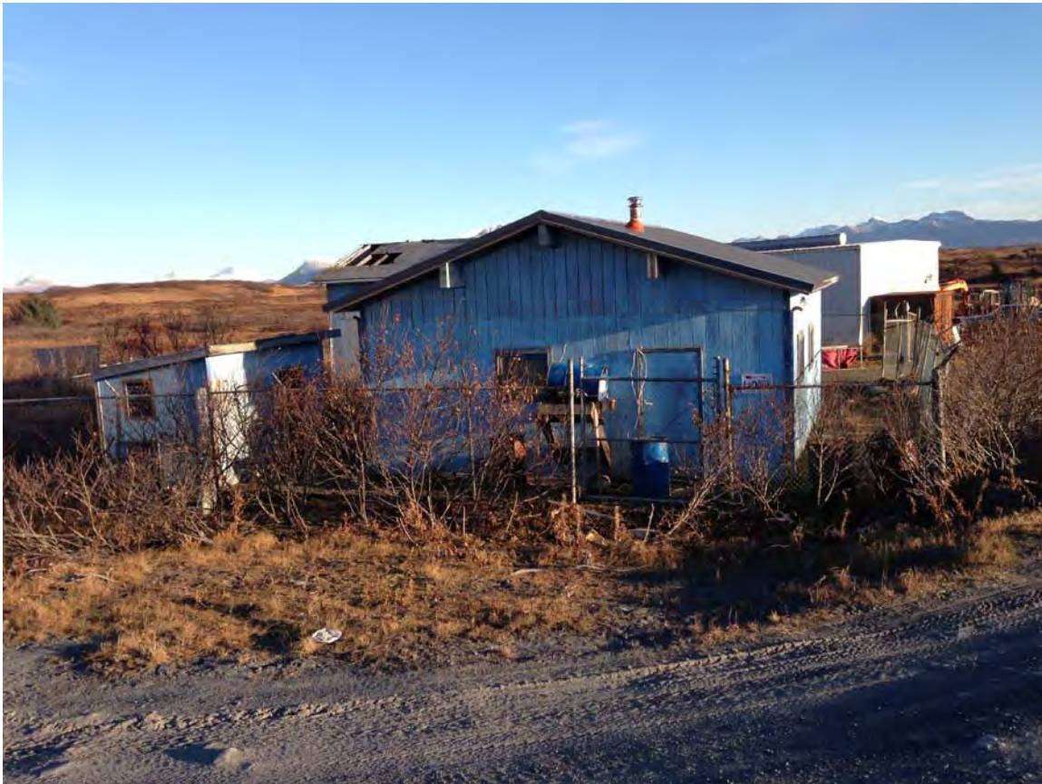
Akhiok's existing WTP
