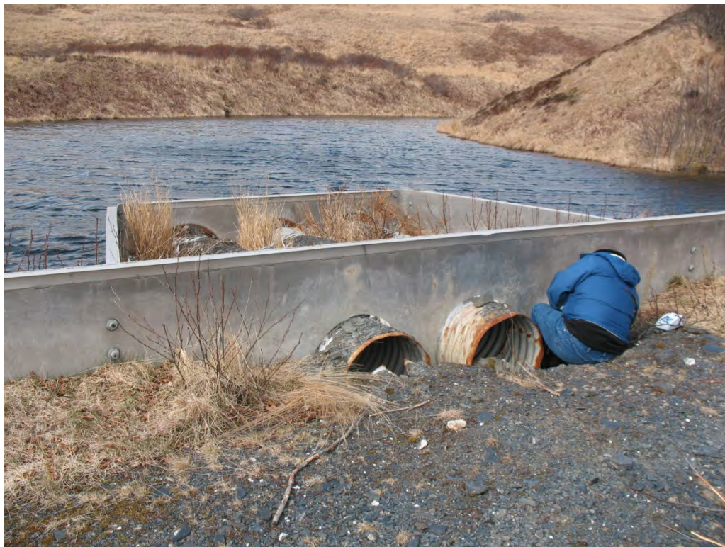
Photograph 4: Intake Structure at source
