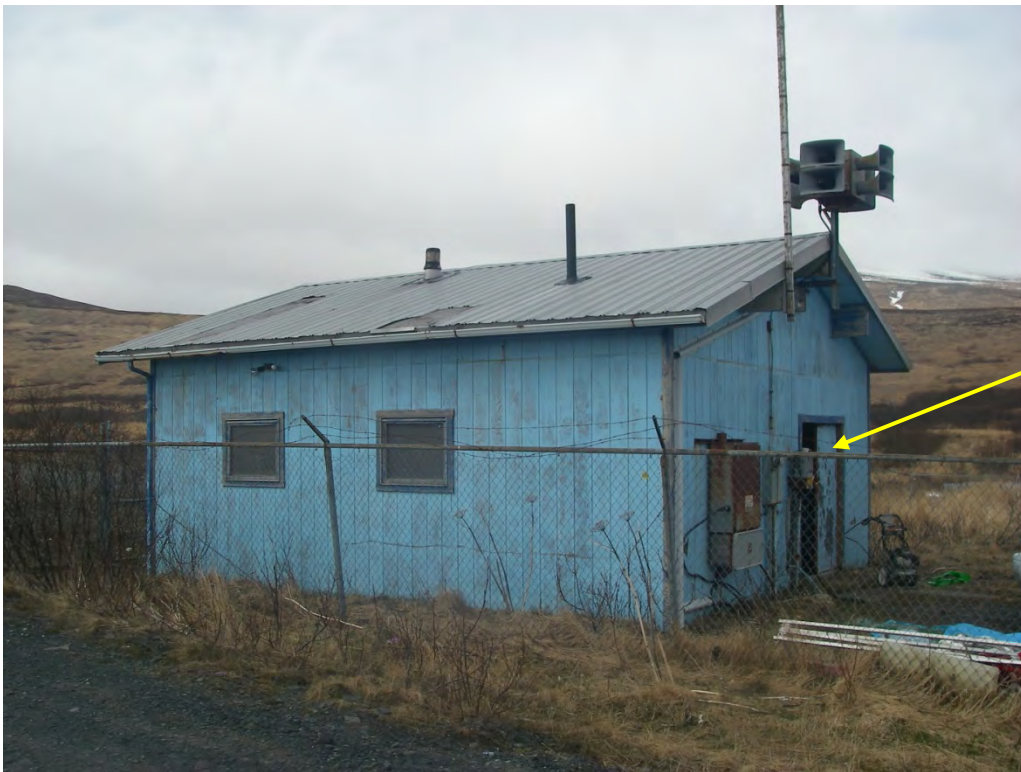
Photograph 2: Water Treatment Plant
