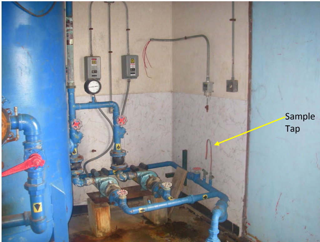
Photograph 5: Raw water sample tap
