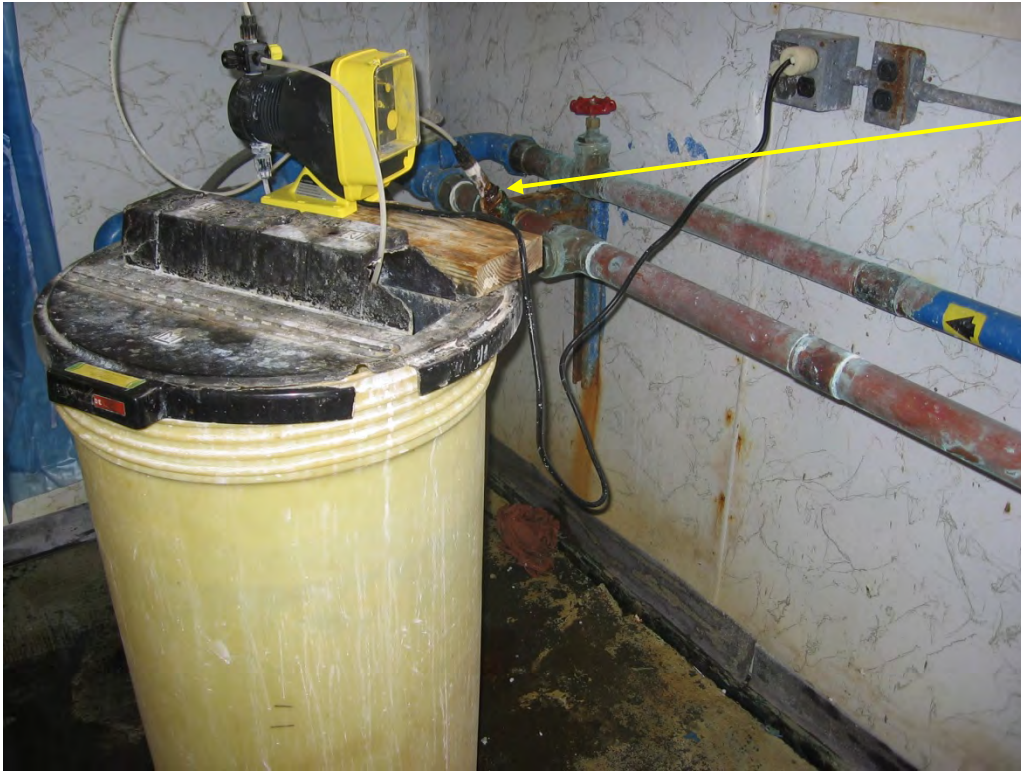
Photograph 7: Chlorine tank and injection point
