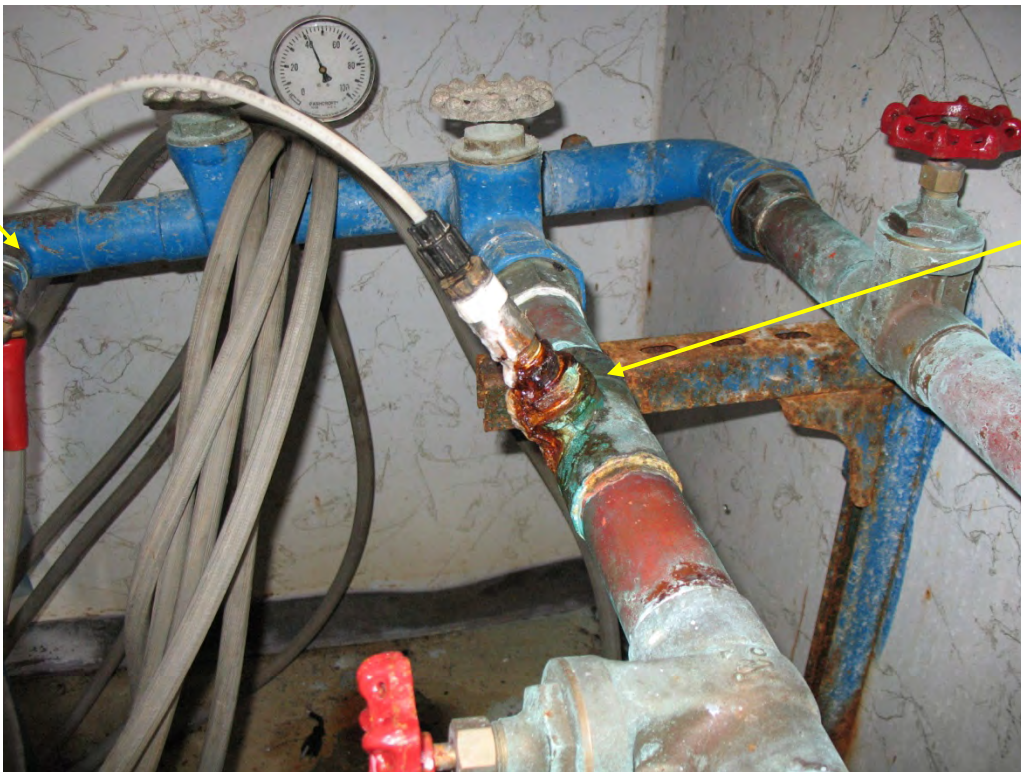
Photograph 8: CFE sample tap (hose)
