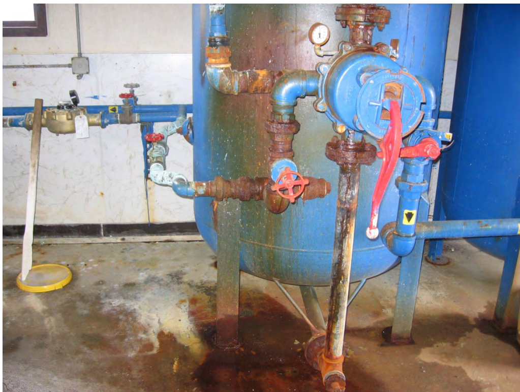
Photograph 6: Working sand filter (left)
